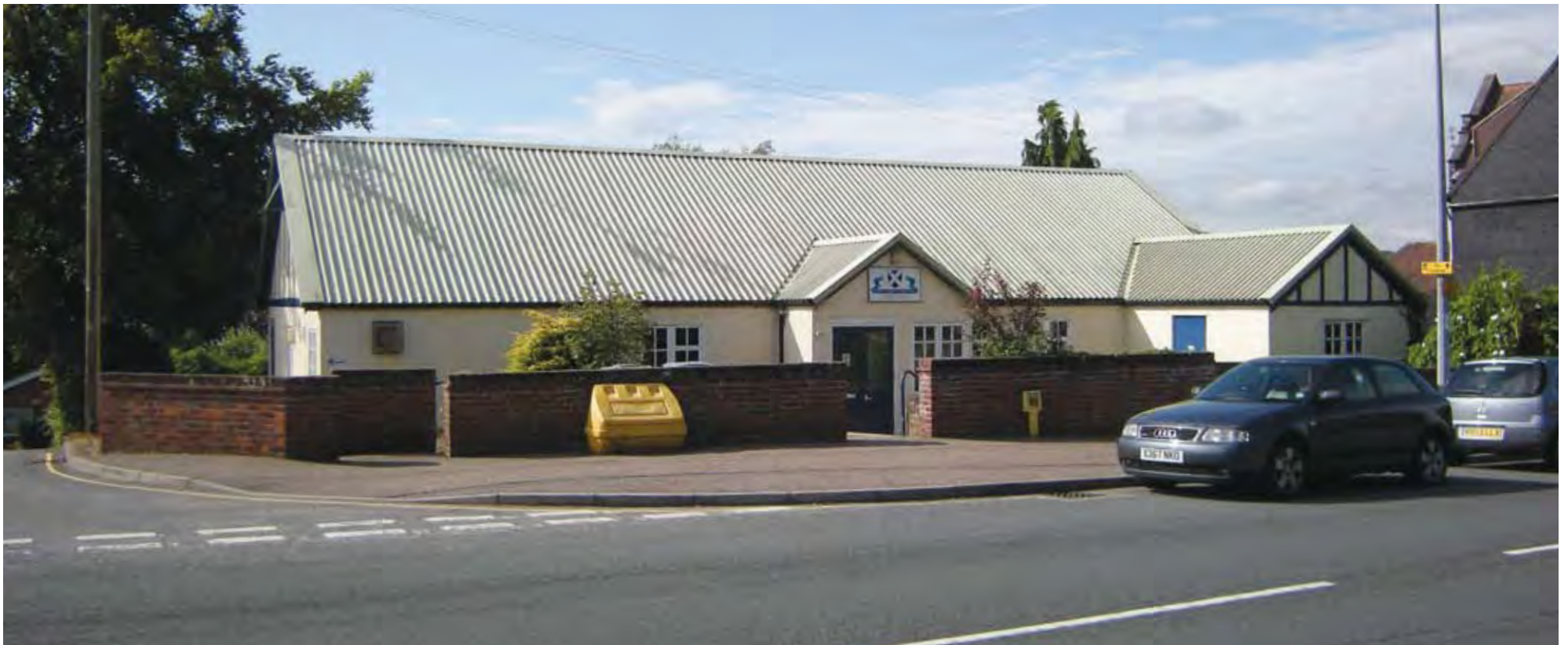
Village Hall, Yarmouth Road
