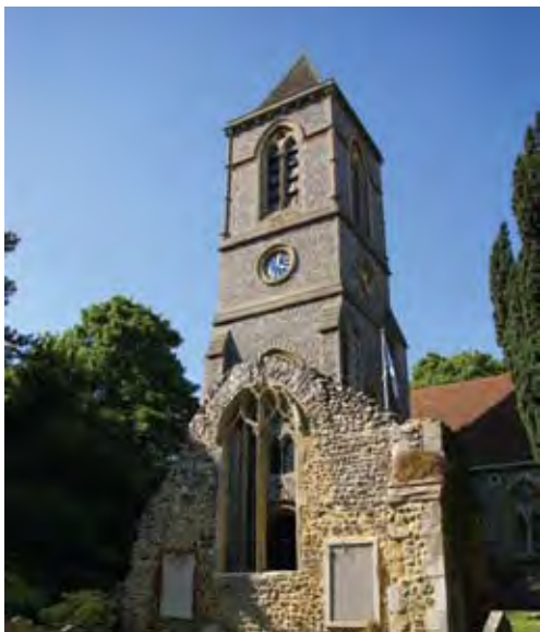
Parish Church, Yarmouth Road
