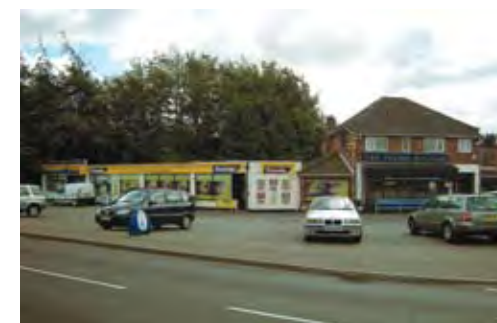
Furze Road Shops
